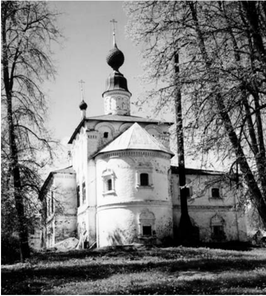
Fig. 14.225. The Church of Presentation, Nikolo-Ouleimenskiy Monastery, Ouglich. Eastern view. A more recent square block topped by a cylinder and also characterised by a semi-circular altar part was adjoined to the old building in some later epoch. Photograph taken in 2000.
